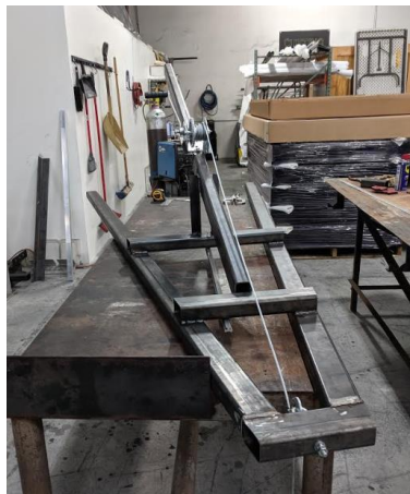
Figure 14. Winch & Pulley Additions
